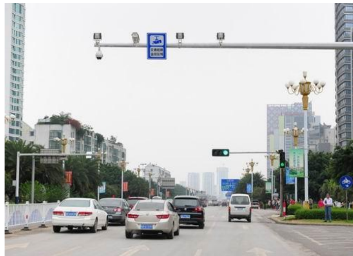
Figure B-7. Traffic Cameras with the Sign Next to Them
